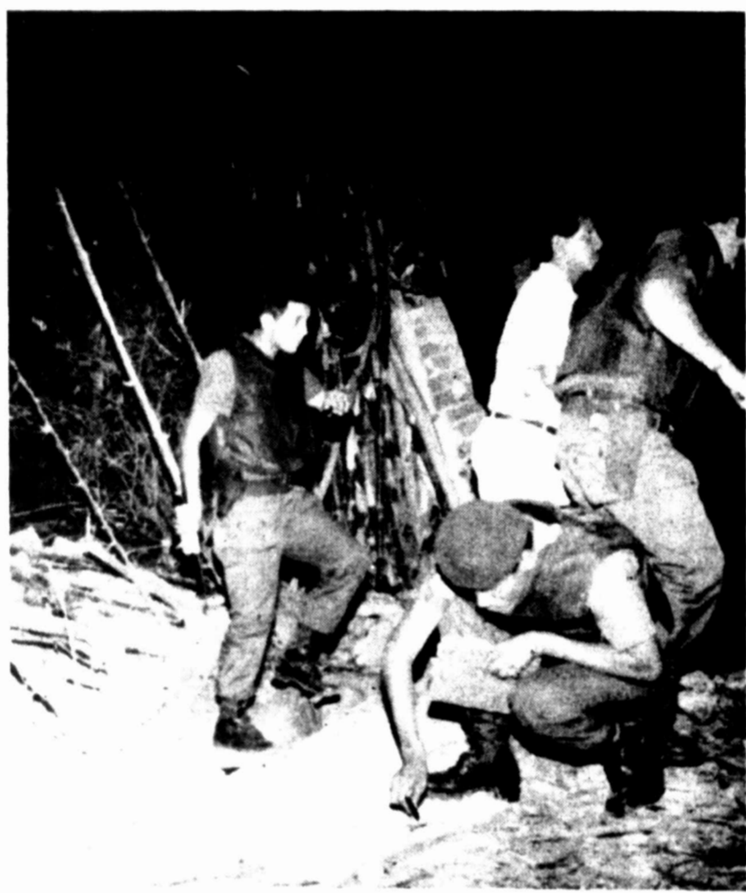
Police pick through the rubble left by a powerful car bomb that exploded outside the U.S. Ambassador's residence in Lima, Peru, Tuesday. The blast damaged a wall behind the building, broke windows, knocked down trees and toppled power lines in the area. Neither of Peru's two leftist rebel groups immediately claimed responsibility for the attack.
