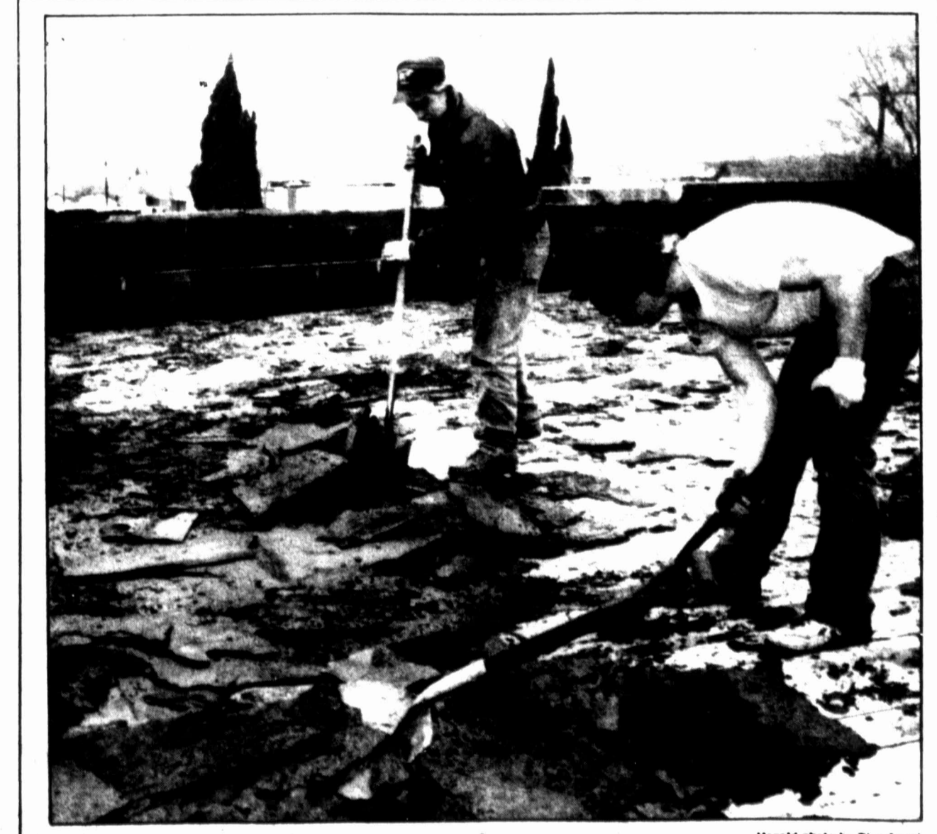
Dig that roof Gerald Buck Jr. and Billy Boulton remove tar paper from the roof of a building in the 1700 block of South Gregg Street Tuesday afternoon. The building is being demolished.
