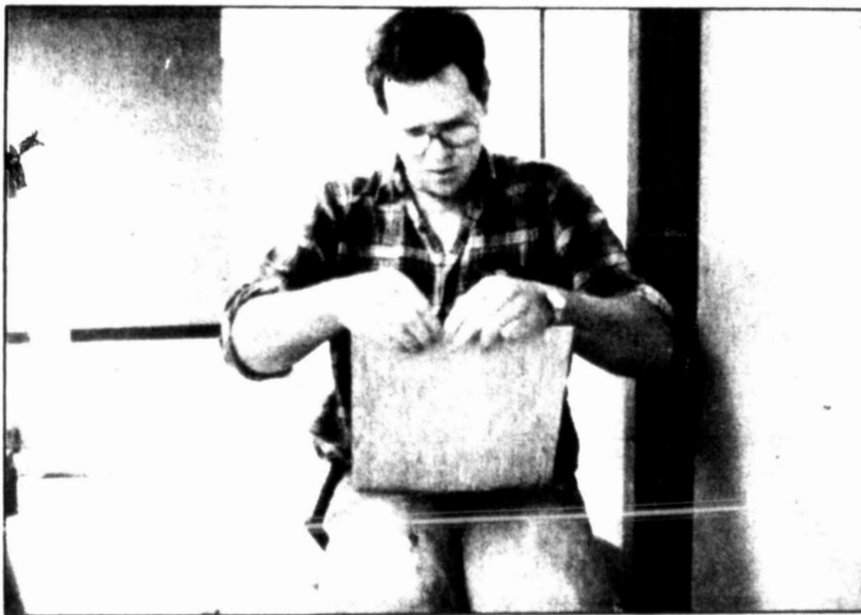
Andy McBee of Brady Floors works on a tile for the second floor of the new Howard County Mental Health Center, 317 Runnels St. The staff will be moving from its current location at the Big Spring State Hospital to the new facility in the first week of February.
