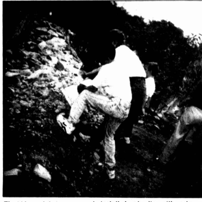
The kids work to cover a newly installed water line with rocks.
