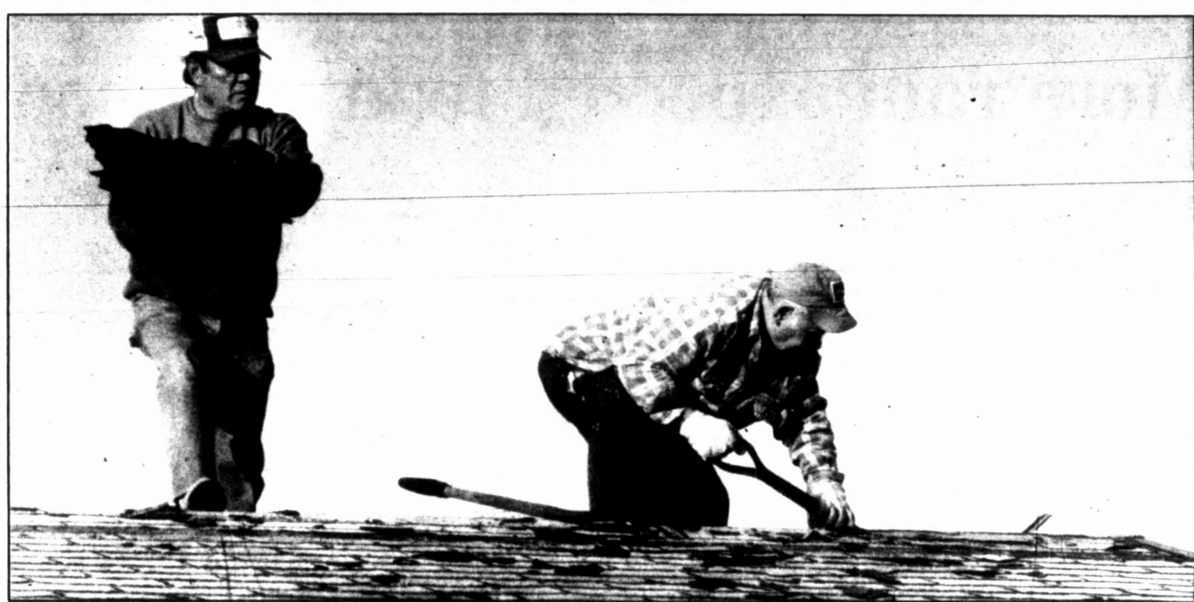
Mickey Renya, left, carries shingles away as H.D. Barber removes them with a pitchfork as the two employees of B&B Roofing were working on a hail-damaged home on Central Drive.
