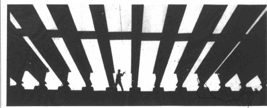
SAN ANTONIO — Tony Martinez of Austin Bridge Co. prepares a safety line on top of what will be a new highway interchange near downtown San Antonio. Concrete plates will be laid on top of the steel beams to form the road's surface.
