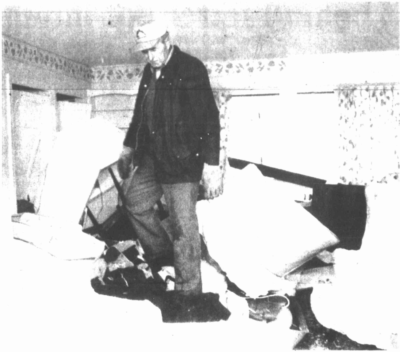
President Bush looks over damage Saturday in a family room of his vacation home on Walker's Point in Kennebunkport, Maine. The Bush compound was hit hard by a severe Atlantic storm Wednesday.
