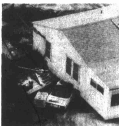
HOME PULLED OFF FOUNDATION
