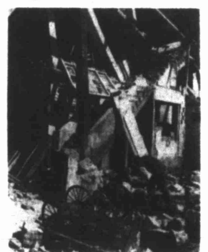
DIGGING THROUGH RUBBLE
