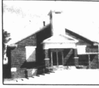
Everything old is new again at the First Baptist Church. The photo on the left is the old front of the church. Above you can see the recently completed new addition.
