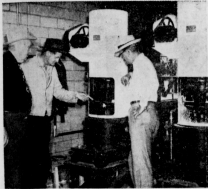
WATER PURIFIED —Mayor B. H. Freeland, W. L. Ray, and C. W. Sutphen, left to right, examine the purifying equipment of Baird's new water system. The agitator at left contains alum and the one at right contains lime. Most of the sediment and other foreign matter is "settled" out of the water by action of the alum and lime.
