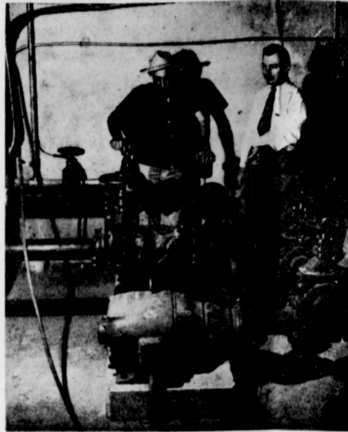
WATER BOOSTED INTO BAIRD —This centrifugal pump takes the water from the filter plant and sends it on its way into Baird for the use of citizens. Examining the pump room are Tom Barton, left, and Marvin Hunter, Baird officials.
