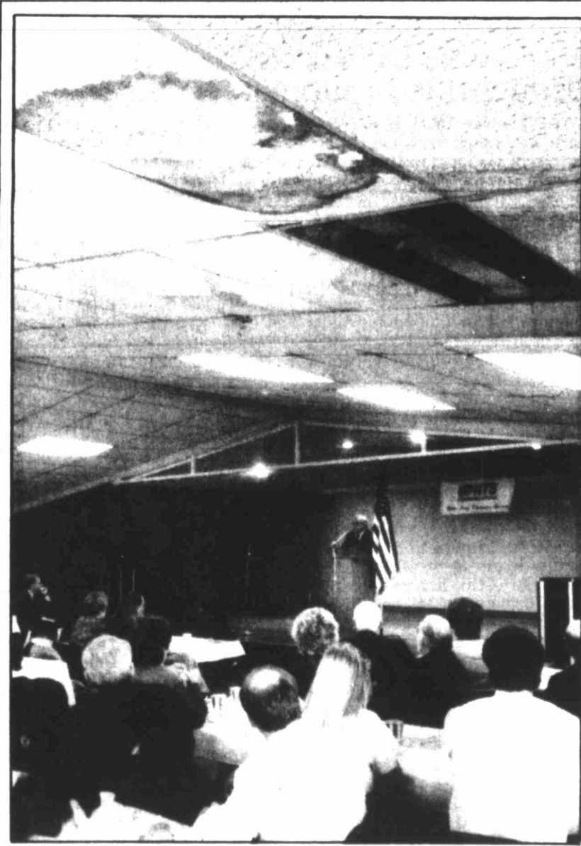
Those in attendance at the Chamber Luncheon Tuesday at the Dora Roberts Community Center sat beneath water-damaged ceiling tiles as Public Works Director Tom Decell talks about renovation plans for the building.
