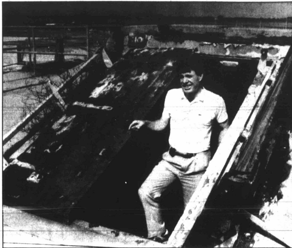
VENUS, Texas — Eric Ducane, the caretaker of a former anti-ballistic missile base near Venus, Texas, poses at the shaft of one of the three underground rooms that once stored missiles.
