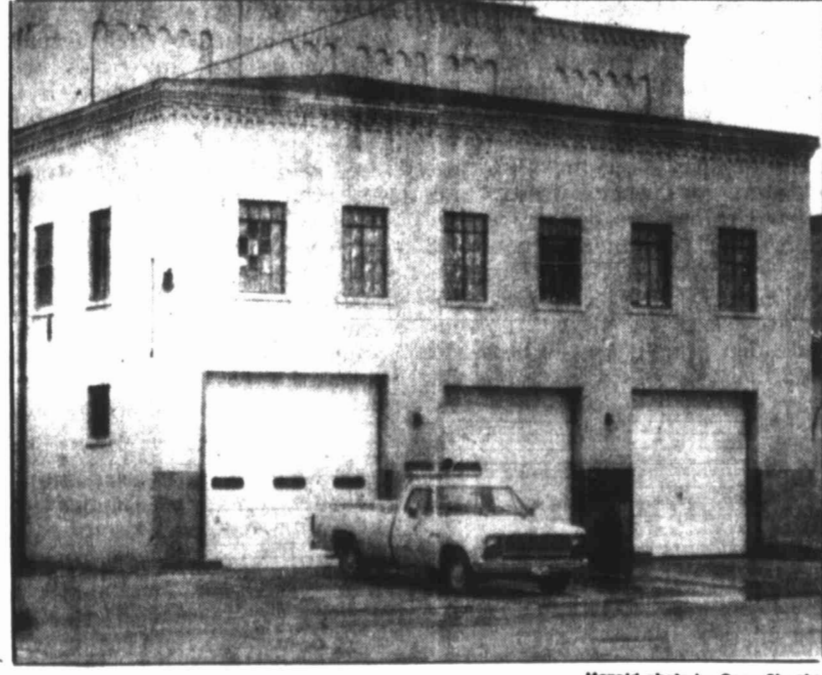
The Central Fire Station at Fourth and Nolan streets is unnecessary, according to a new study. Overlapping coverage of stations two, three and four create redundancy in fire protection for the city, the report said.
