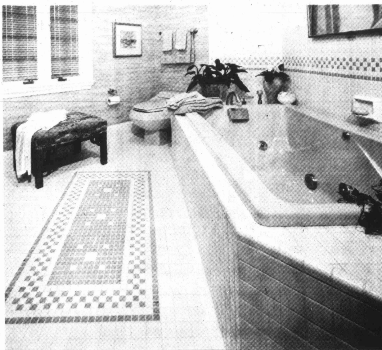
Designs with ceramic tile can take any shape imaginable. In this charming room, bathers can step out onto a "rug" of 2" x 2" unglazed ceramic mosaics surround by 2" glazed ceramic mosaics.
