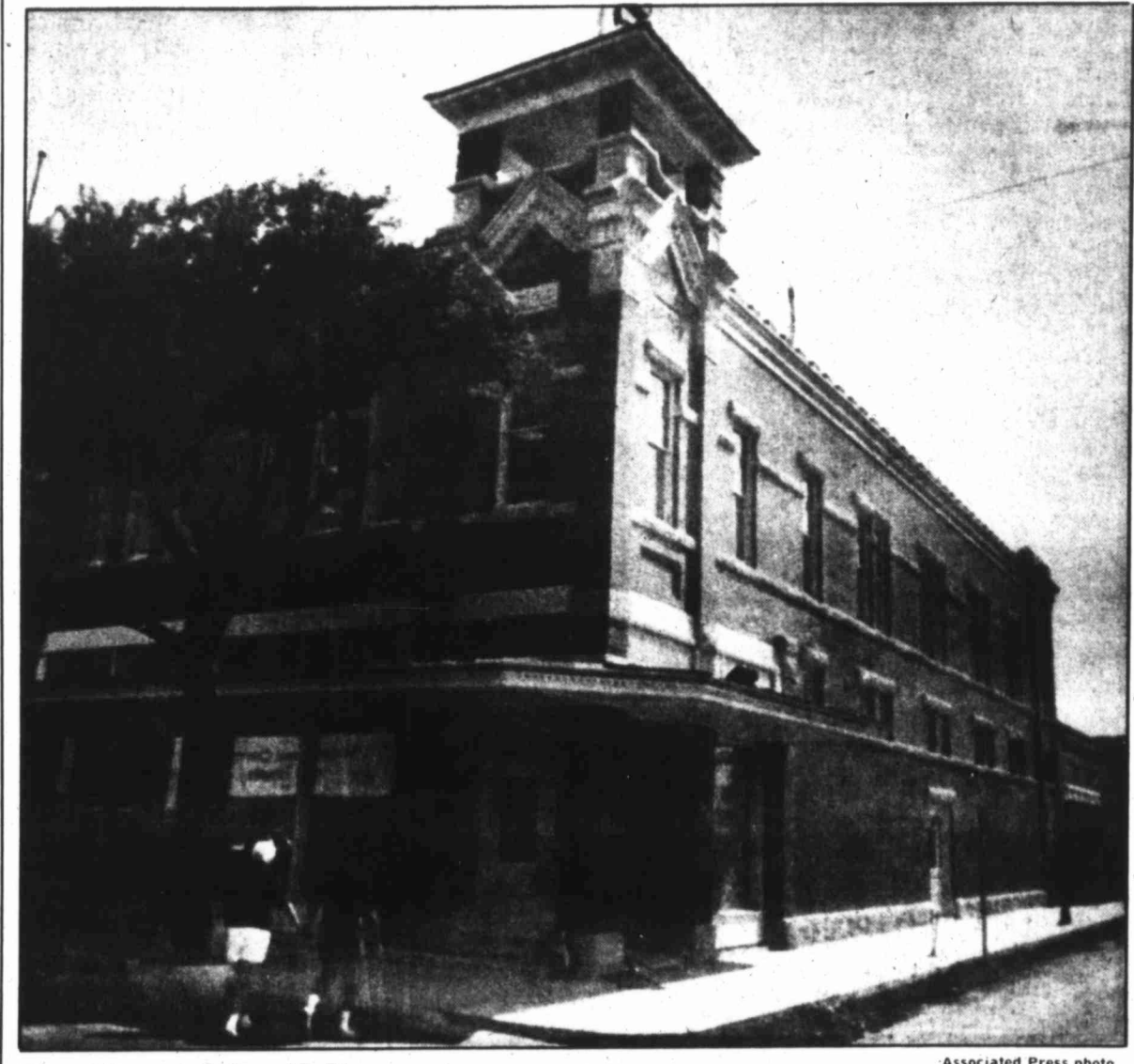
Restored building KINGSVILLE — The Ragland Building, formerly known as Ragland's Department Store, at the corner of Sixth Street and Kleberg Avenue in Kingsville has recently been restored by the King Ranch. The store, originally opened in 1909 as the John B. Ragland Mercantile Co., will open Saturday as King Ranch Saddle Shop.
