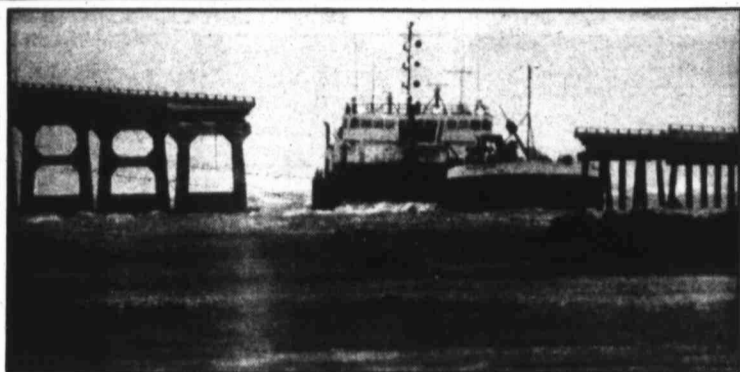
BONNER BRIDGE TOPPLES
