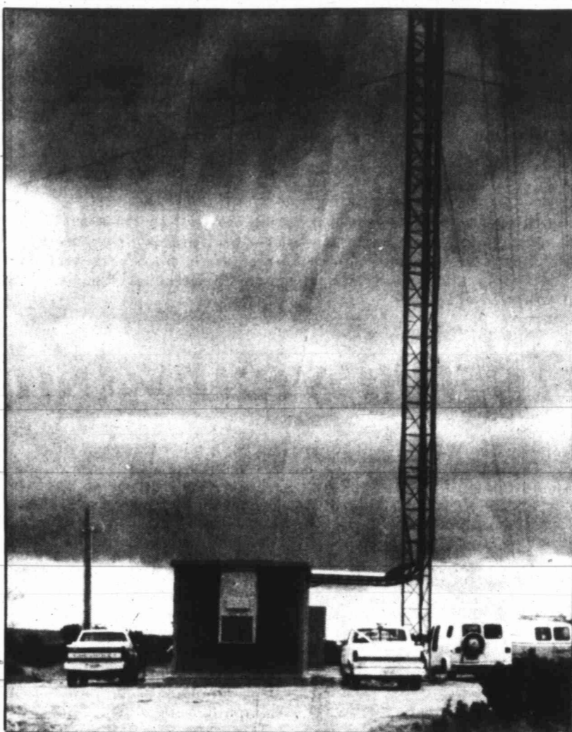
Westex Telecommunications of Stanton has erected a 480-foot cell tower south of Big Spring for its upcoming cellular telephone service in this area. Westex anticipates beginning cellular service sometime around mid-October.
