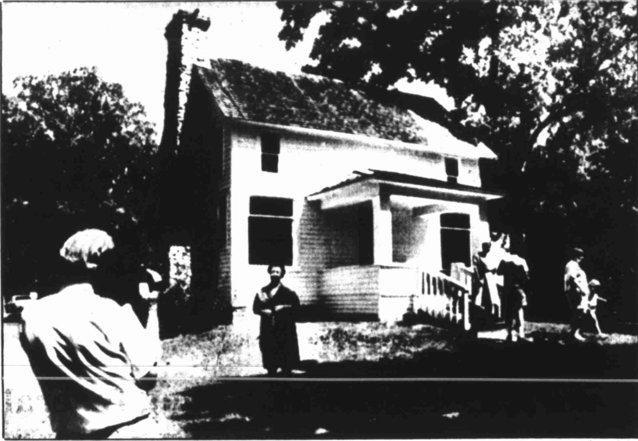
Little house MANSFIELD, Mo. — Author Laura Ingalls Wilder and her husband, Almanzo, lived in this home near Mansfield in Missouri's Ozarks for more than 50 years after leaving South Dakota in August, 1894. Laura wrote "Little House on the Prairie" and 10 other best-selling children's books while living in this house.
