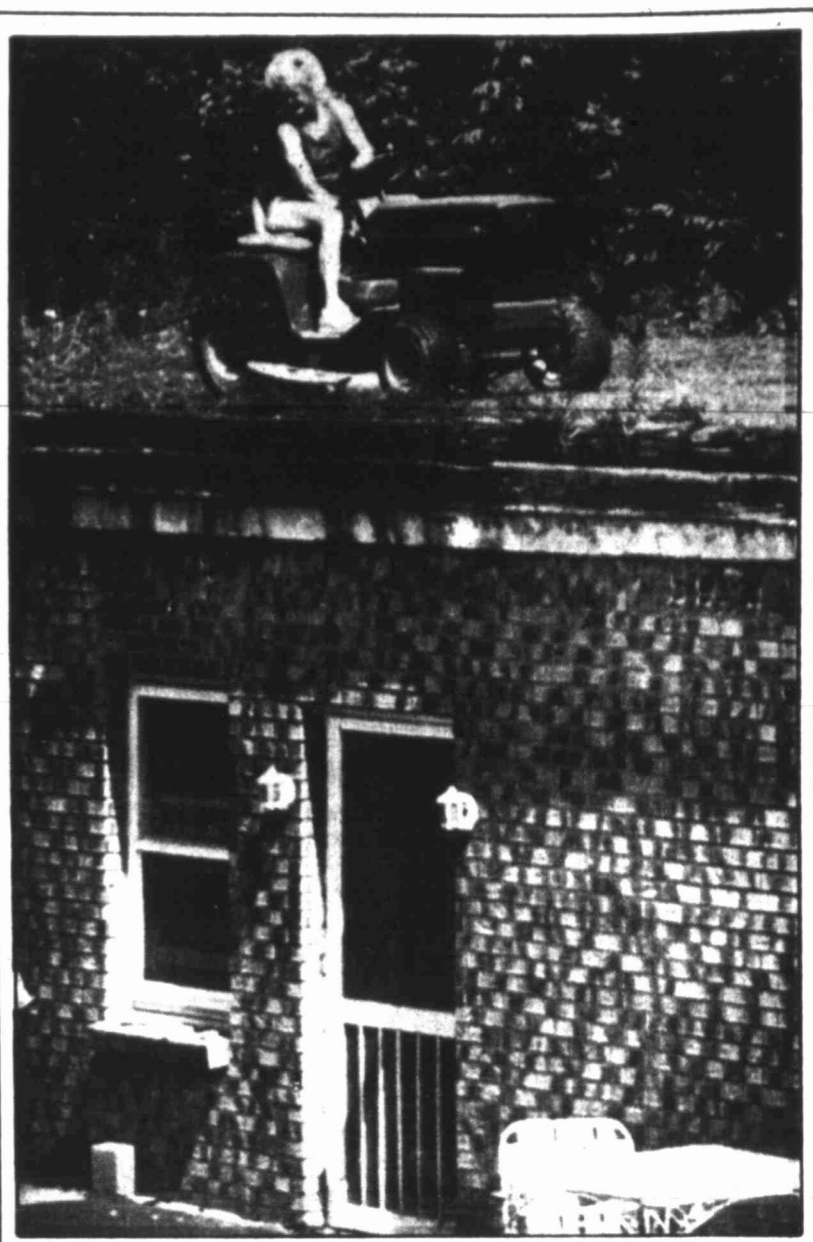
A little off the top LAFAYETTE, N.Y. — Suzanne Dodge takes lawn mowing to a higher plane as she cuts the grass on the roof of her Lafayette, N.Y., home Monday. The house is built into the side of a hill to save energy, and has rooms that extend five feet underground, in addition to grass on the roof.
