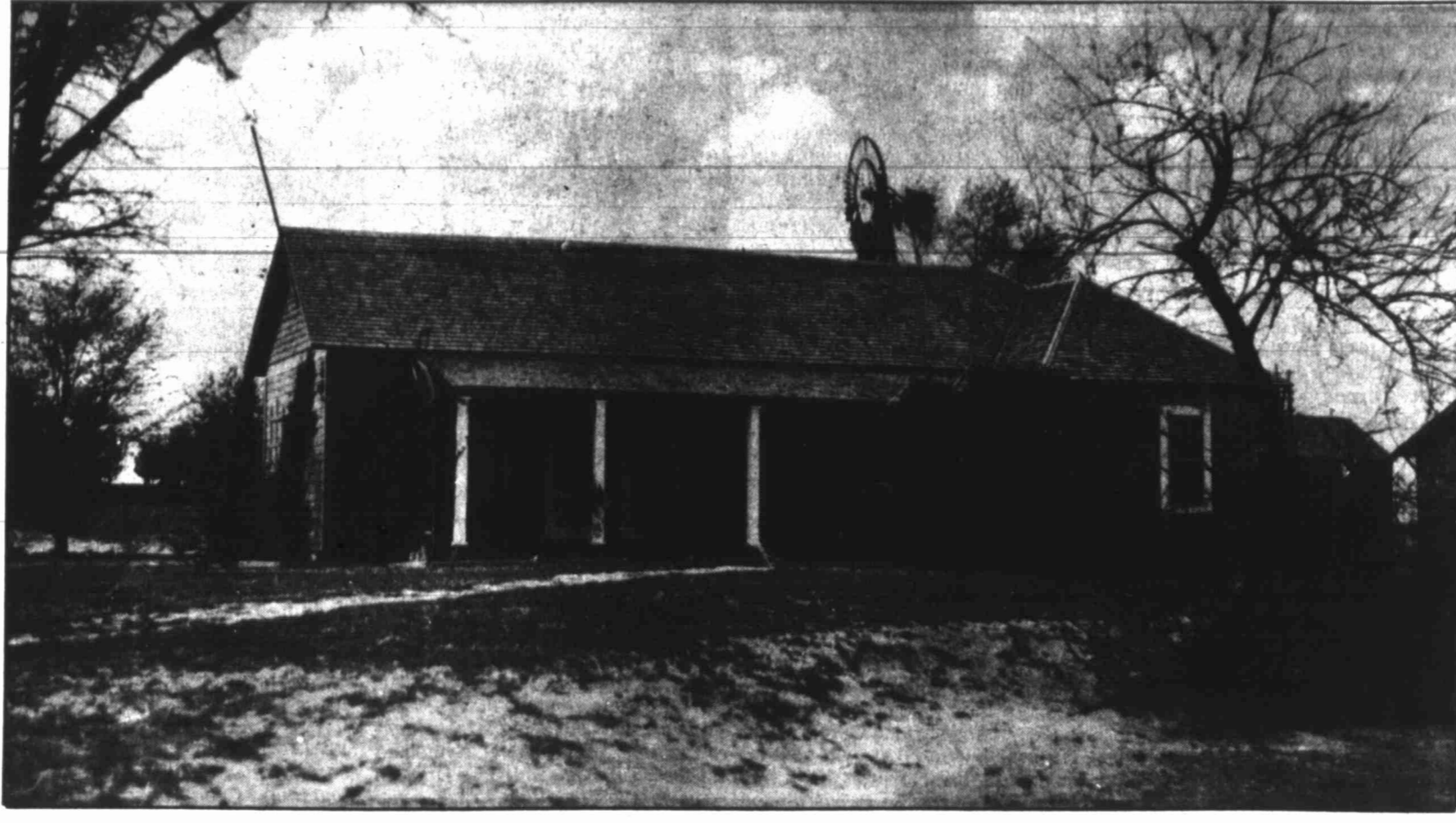
The original two rooms of the Connell family homeplace at 410 Convent St. is probably the oldest structure in Stanton. When the last
