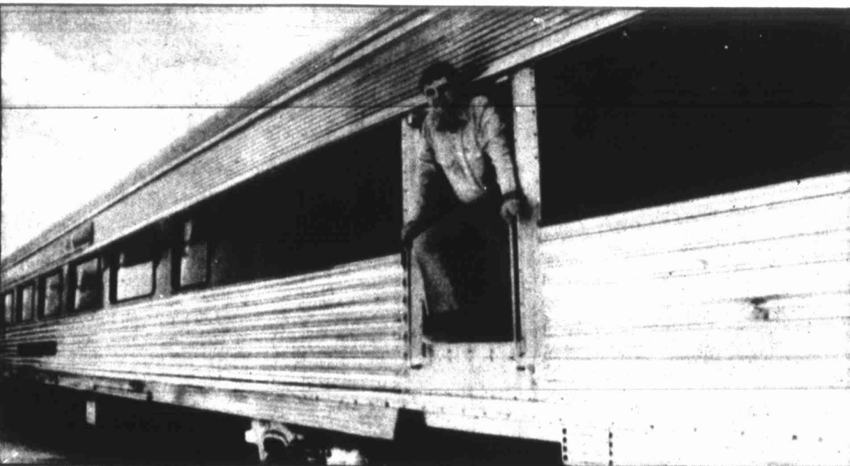
AUSTIN — Joe Pinelli leans out of the railroad car he restored for use as an excursion train between Galveston and Houston. The car arrived without doors, windows or lights, which had to be manufactured to original specifications.
