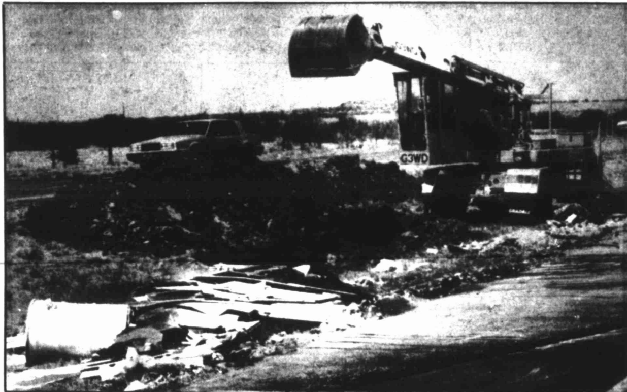
A damaged 18-wheeler, above, hit the back of a paint striping truck on June 29. Cleanup operations included burying more than 500 pounds of debris from the accident. Some of the material should not have been buried there, state officials said.
