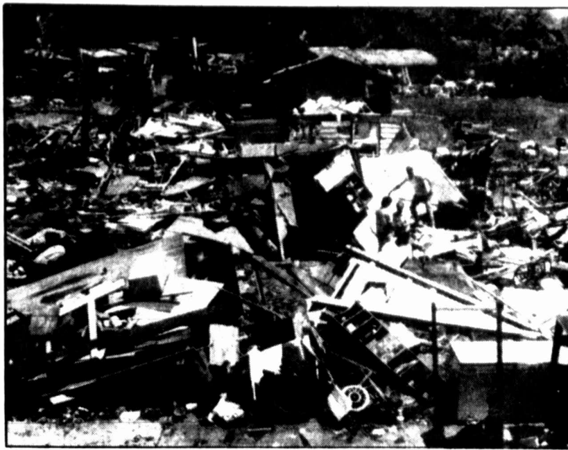
HARRISON, Ohio — Residents sift through the remains of several homes leveled by a tornado late Saturday night in Harrison, Ohio.
