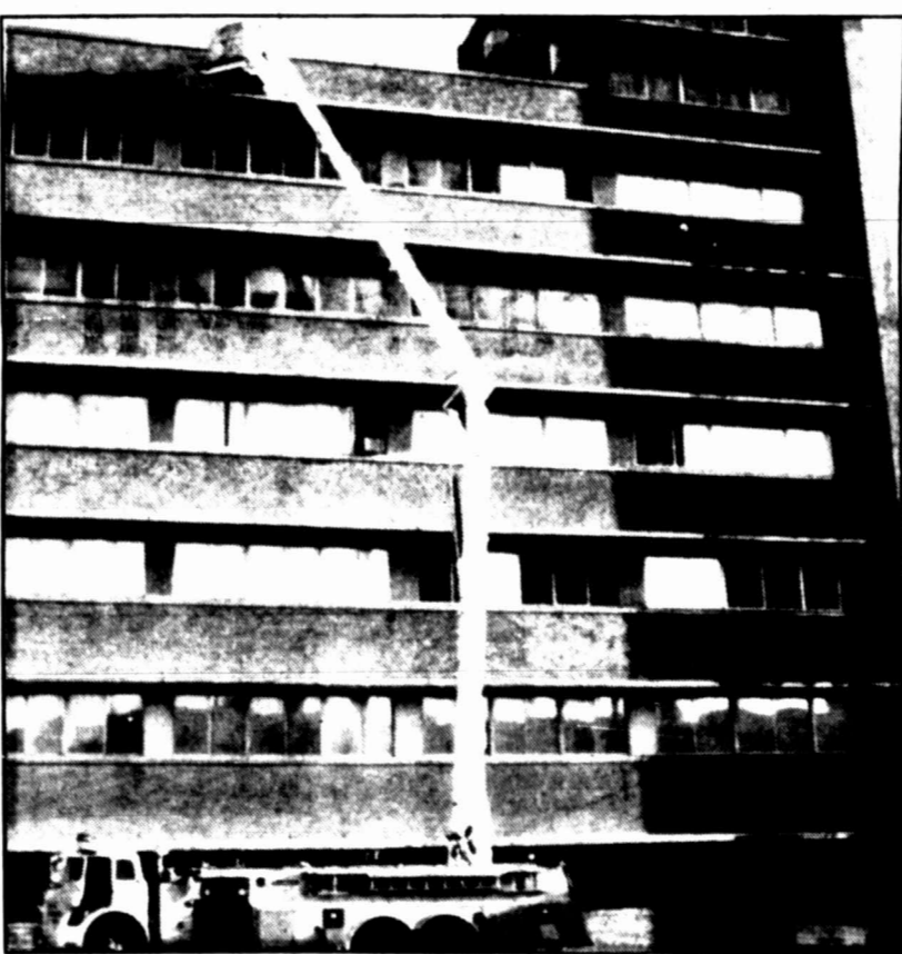
BIG SPRING — Fire fighters were called to the Permian Building early this morning after a fire was reported in the penthouse. The blaze apparently was caused by electricity. The fire is the latest in a series of mishaps, including a broken water pipe that has caused several tenants to move from the building.
