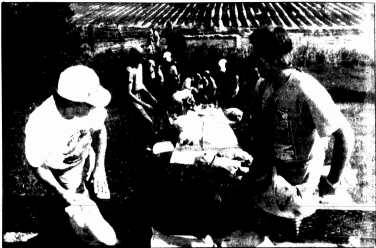
GARLAND, Ark. — Hundreds of volunteers turned out in Garland, Ark., to help sandbag areas of the levee where Army Corps engineers spotted seepage. A Texas National Guard helicopter airlifted the sandbags to the levee and volunteers transported them to the areas where needed.
