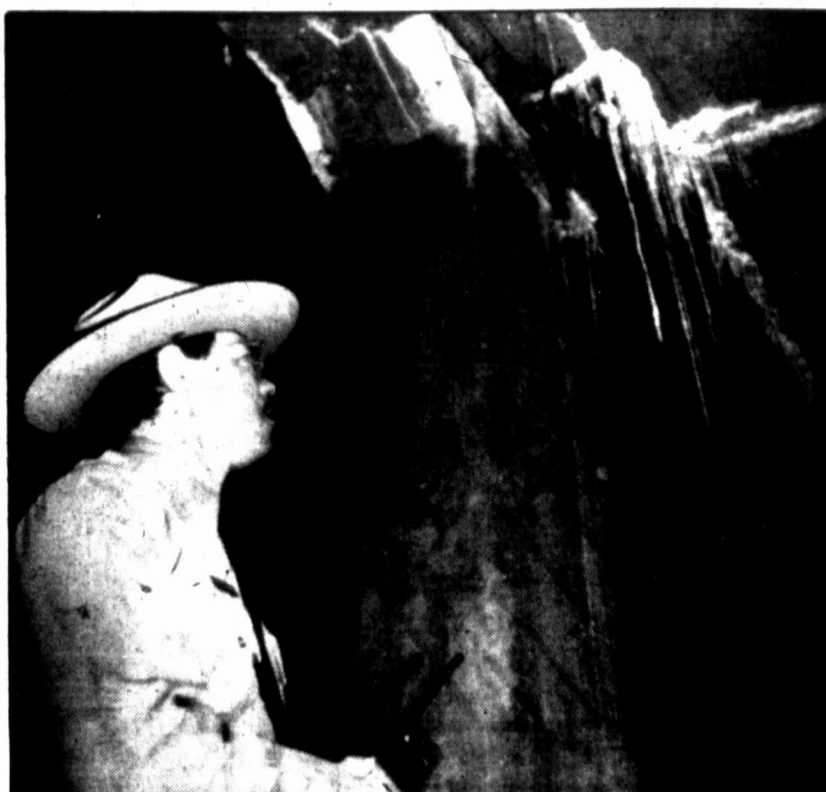
WASHINGTON — National Park Service ranger John Hannan looks at some of the stalactites hanging from cracks and joints in the ceiling of the Lincoln Memorial in Washington last week.
