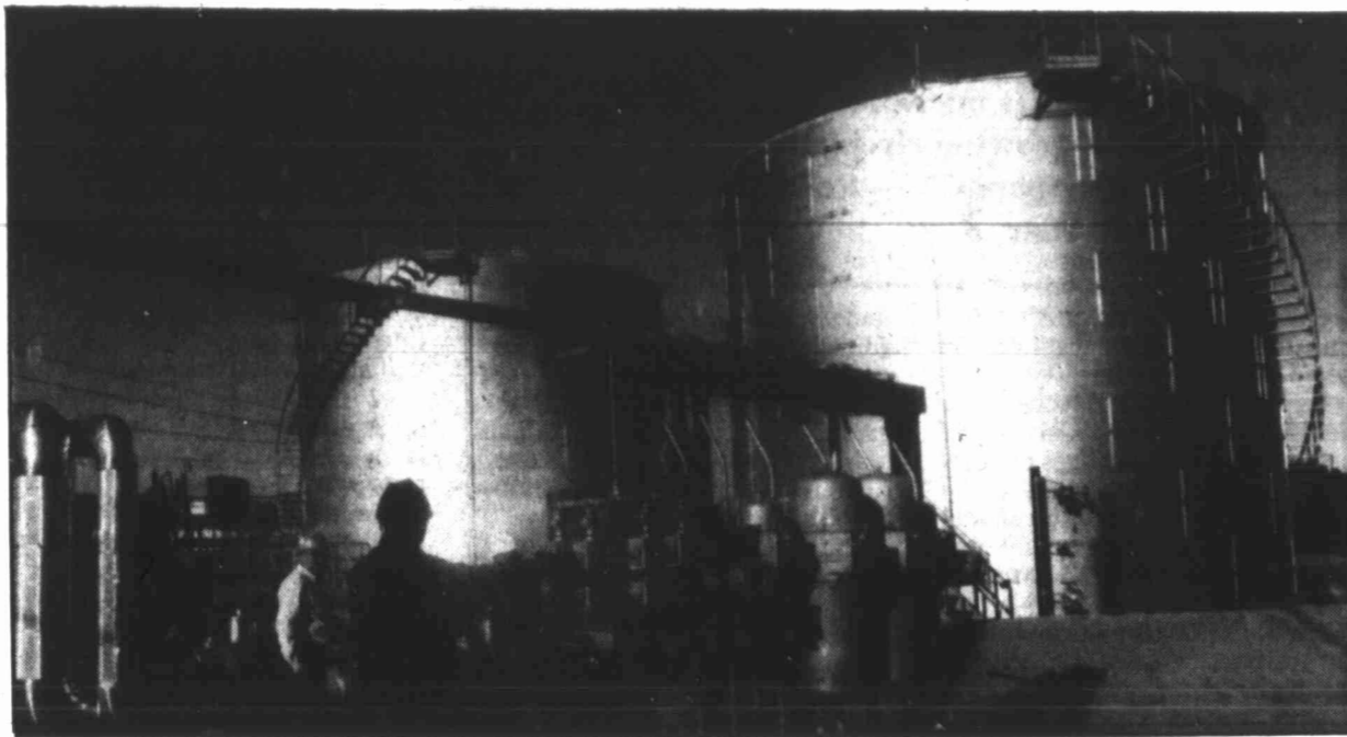
BIG SPRING — Two storage tanks will go on line this week for use in loading asphalt onto railroad cars at the Fina Refinery.
