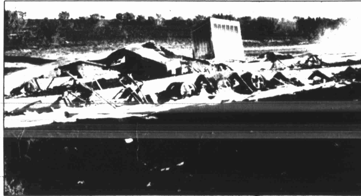
Firefighters examine wreckage of a mobile home, top photo, after a Sunday afternoon fire destroyed the home, which is in the Tubbs addition. Another mobile home, bottom photo, also caught fire and was destroyed. Investigators said the blaze started after sparks from an acetylene torch caught the first home on fire. Eight fires ravaged the Crossroads area Sunday.
