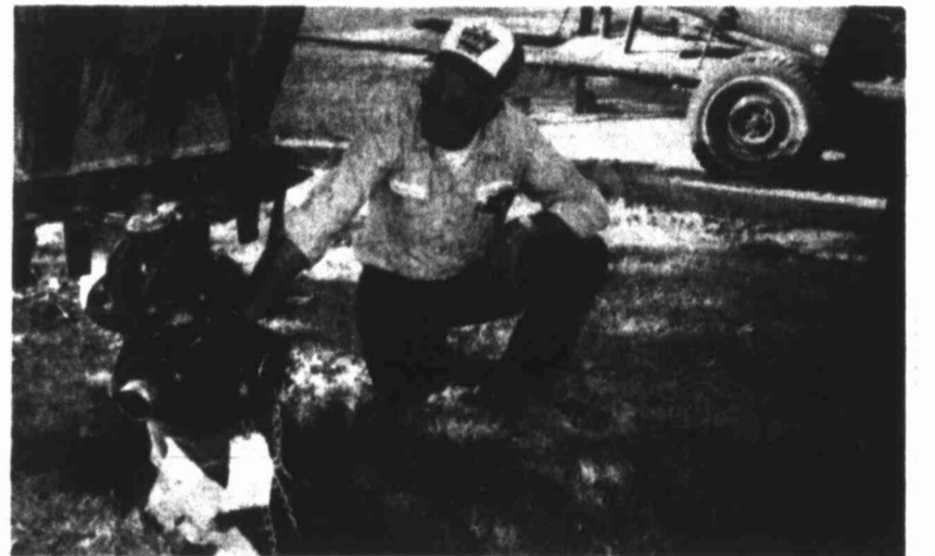
Robert Helm of the City of Coahoma Water Dept. inspects a new fire plug ready for installation. Areas of the southside of town is undergoing waterline replacement under a 1987 grant the city was awarded.
