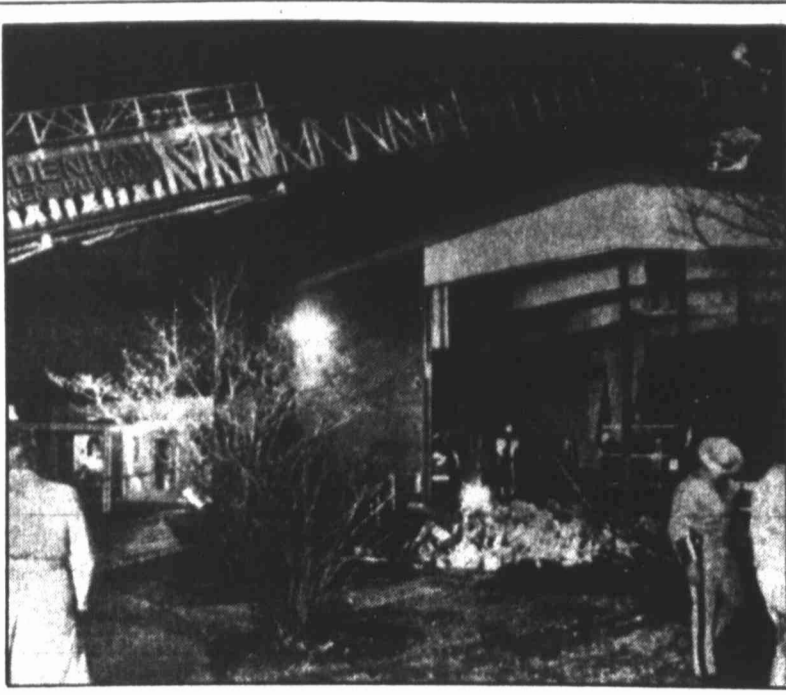
Storm destruction NEWBURGH, N.Y. — A concrete wall of a school cafeteria in Newburgh, N.Y. collapsed Thursday, killing seven children and injuring several others.
