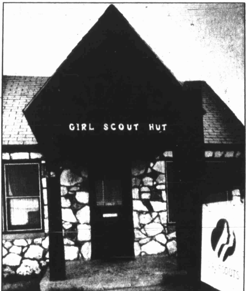
The Girl Scout Council recently remodeled this building at 1609 Scurry Street for scout activities and meetings.
