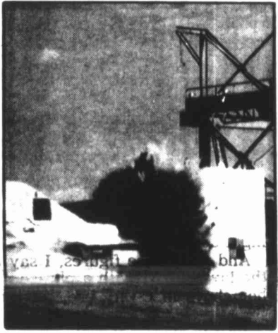
CRASH SCENE 1988. The rocket-propelled F-4 smashed head-on into a 1 million-pound concrete barrier. It shattered when it hit the 23-foot-square, 12-foot-thick reinforced concrete block at 480 mph.
