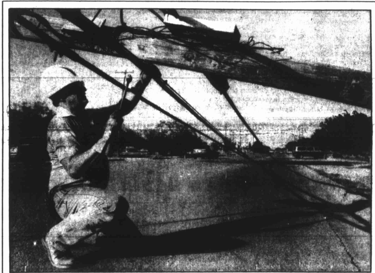
Southwestern Bell employee James Powell kneels beneath one of the downed telephone poles, preparing to remove one of the phone lines after an accident Tuesday.
