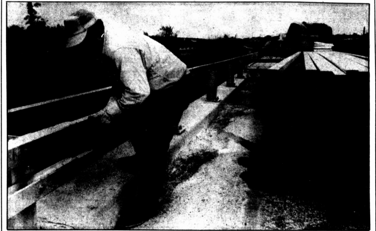
Strickland and Knight employee Leon Molina places a metal connector into one end of a guardrail as a new rail was being installed on the Beals Creek bridge on FM 700 Wednesday morning.
