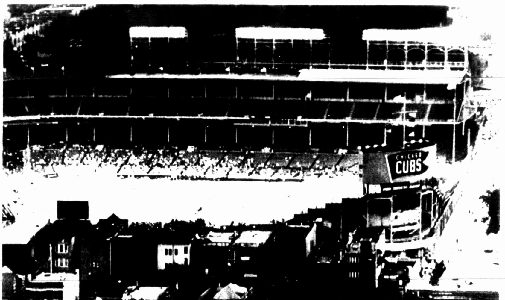
CHICAGO — Light streams from three banks of lights as the Chicago Cubs held their first night practice July 25 at Wrigley Field. Twenty-six panels on six stands were built by General Electric Co.
