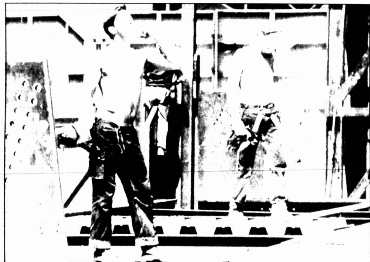
NEW YORK — Two construction workers sweat it out on the job at a Manhattan building site Wednesday as record heat continues to blast New York and the rest of the country. Temperatures this week are expected to near 100 degrees.
