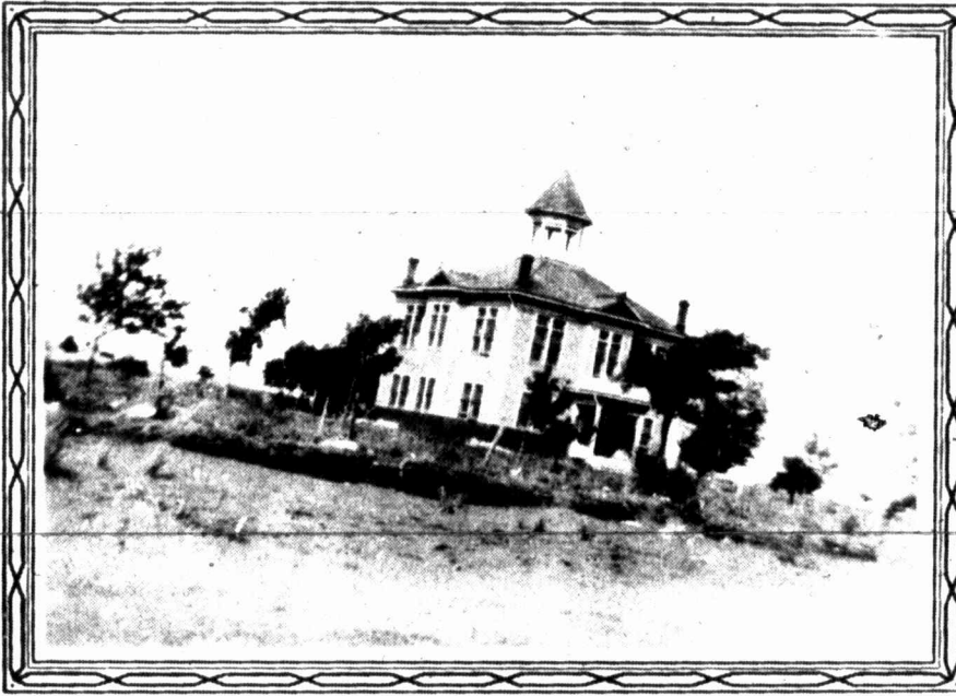
ANDREWS COURTHOUSE — The Andrews County Courthouse about 1929, when Bryan was sent to Andrews by TESCO.
