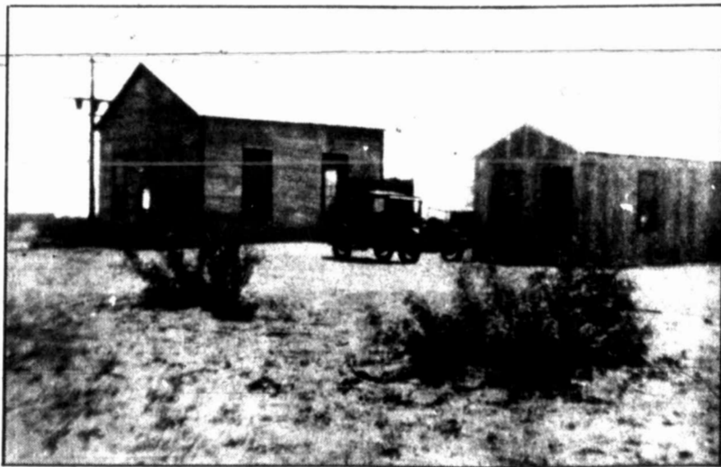
NEXT DOOR — The Andrews TESCO power plant, with the office built later next door.
