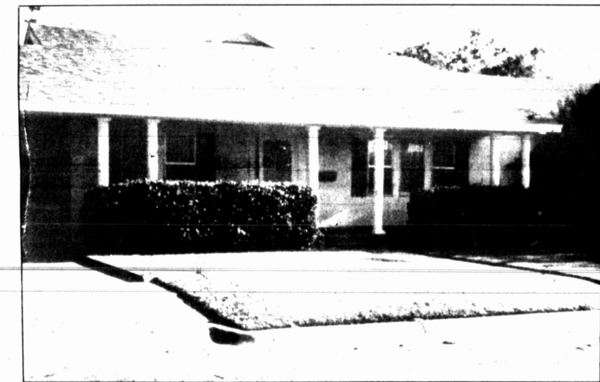
Bob's Custom Woodwork transformed this home in Edwards Heights, giving it a formal exterior with Southern charm. The house roofline, flat porch roof and attached carport roof were all incorporated into one roof, giving the house a more pleasing architectural design. The addition of plantation columns was the final touch.
