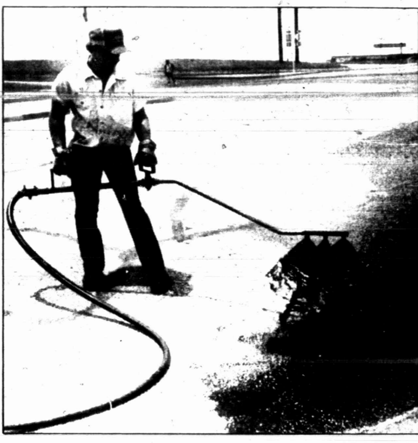
Applying the seal Danny Basham sprays a layer of sealcoating onto the Owens Street turnoff on the south service road of Interstate 20 Wednesday afternoon. The project of sealcoating major highways and Farm-to-Market roads are being done by the Texas State Department of Highways and Public Transportation.
