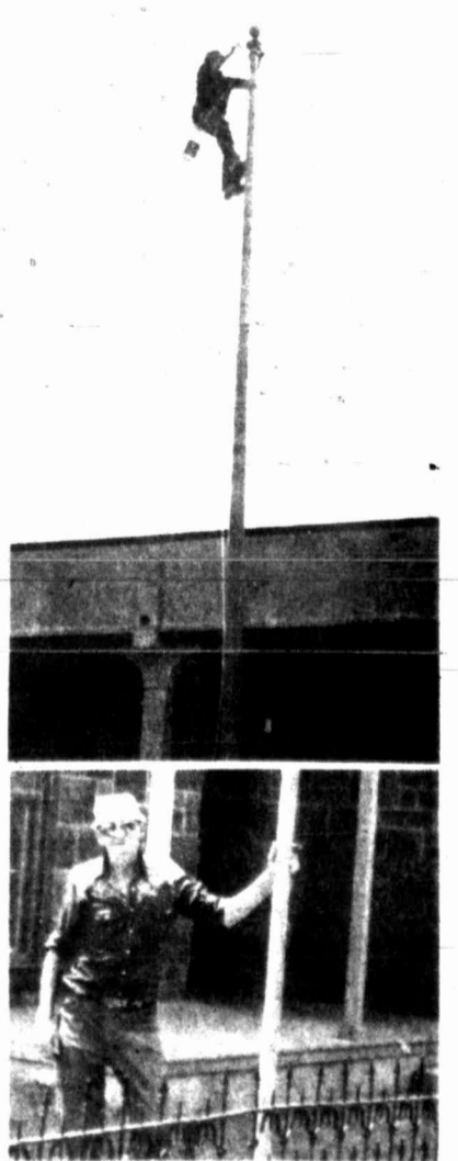
(Photo by Roy Lee Barnhill) FLAGPOLE PAINTER — Sam Gillette, 57, calls Shawnee, Okla., home. However, he goes from town to town painting flagpoles. He is shown above painting one of four flagpoles owned by Martin County. Sam also painted a flagpole owned by First National Bank.
