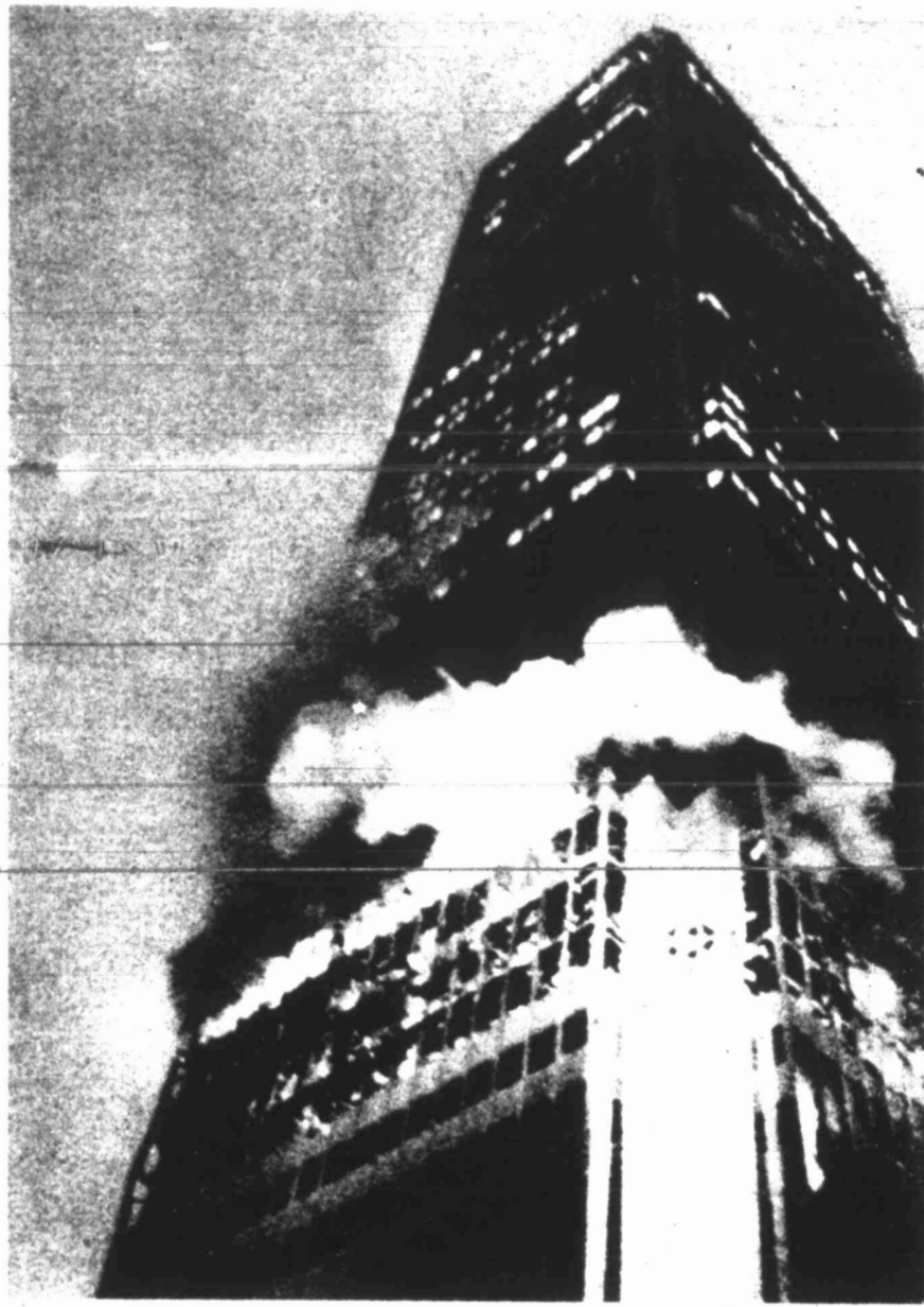
LOS ANGELES — A helicopter soars around the First Interstate building, at left, while flames shoot from the windows of the 62-story building early Thursday morning in downtown Los Angeles. Eight people were rescued from the building by helicopter.
