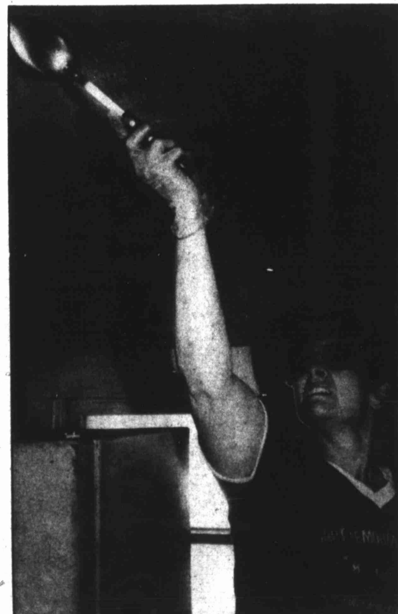
Kay Clark uses a long-handled metal spoon to scrape loose paint from the kitchen ceiling at 810 N.W. 4th Street before a new coat of paint is applied.
