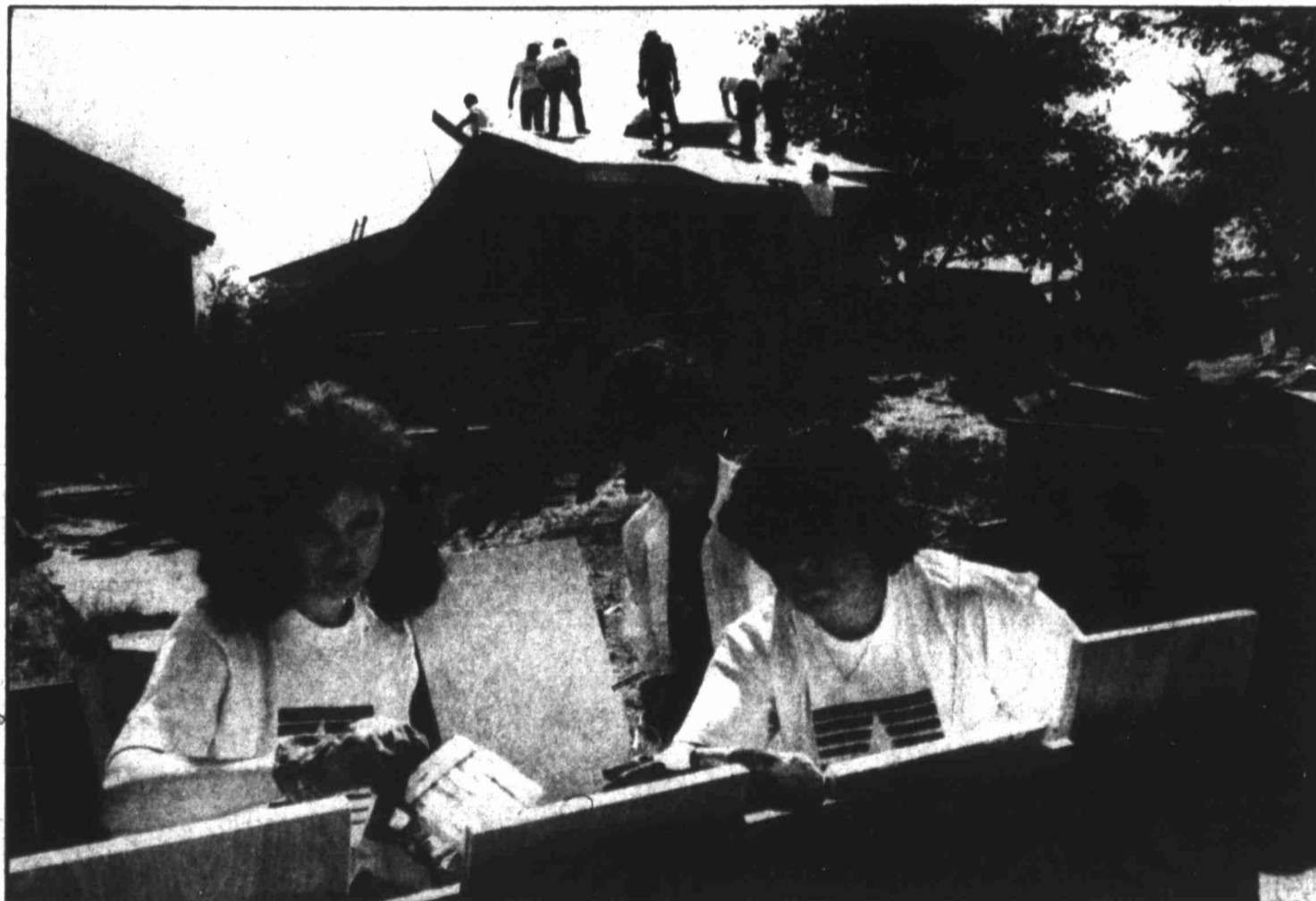
Cheryl Stevens, left, Clara Grimes and Merlinda Chavez paint cabinet doors in a trailer, out of the way from other action as workers from T.U. Electric work on their project house at 508 N. San Antonio.
