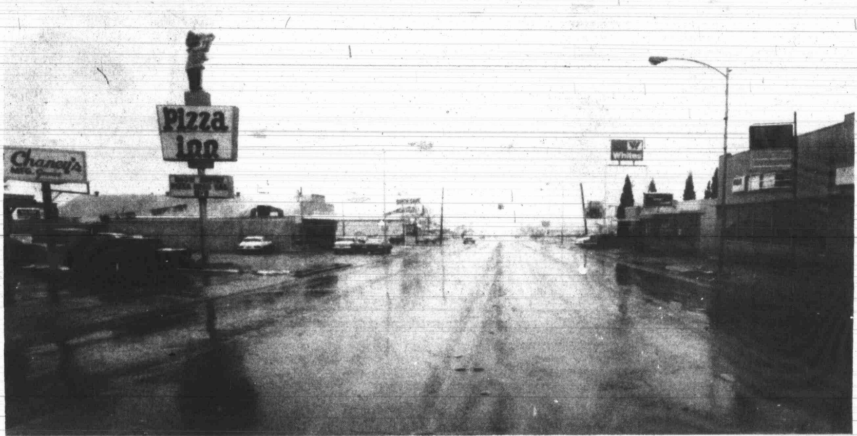
This photo provides a glimpse along a Gregg Street that has been targeted by the state highway department for widening seven feet on both sides for installation of a center left-hand turn lane. The proposal calls for 17 blocks to be expanded, from FM 700 to 10th Street using $750,000 in state funds. State highway depart-
