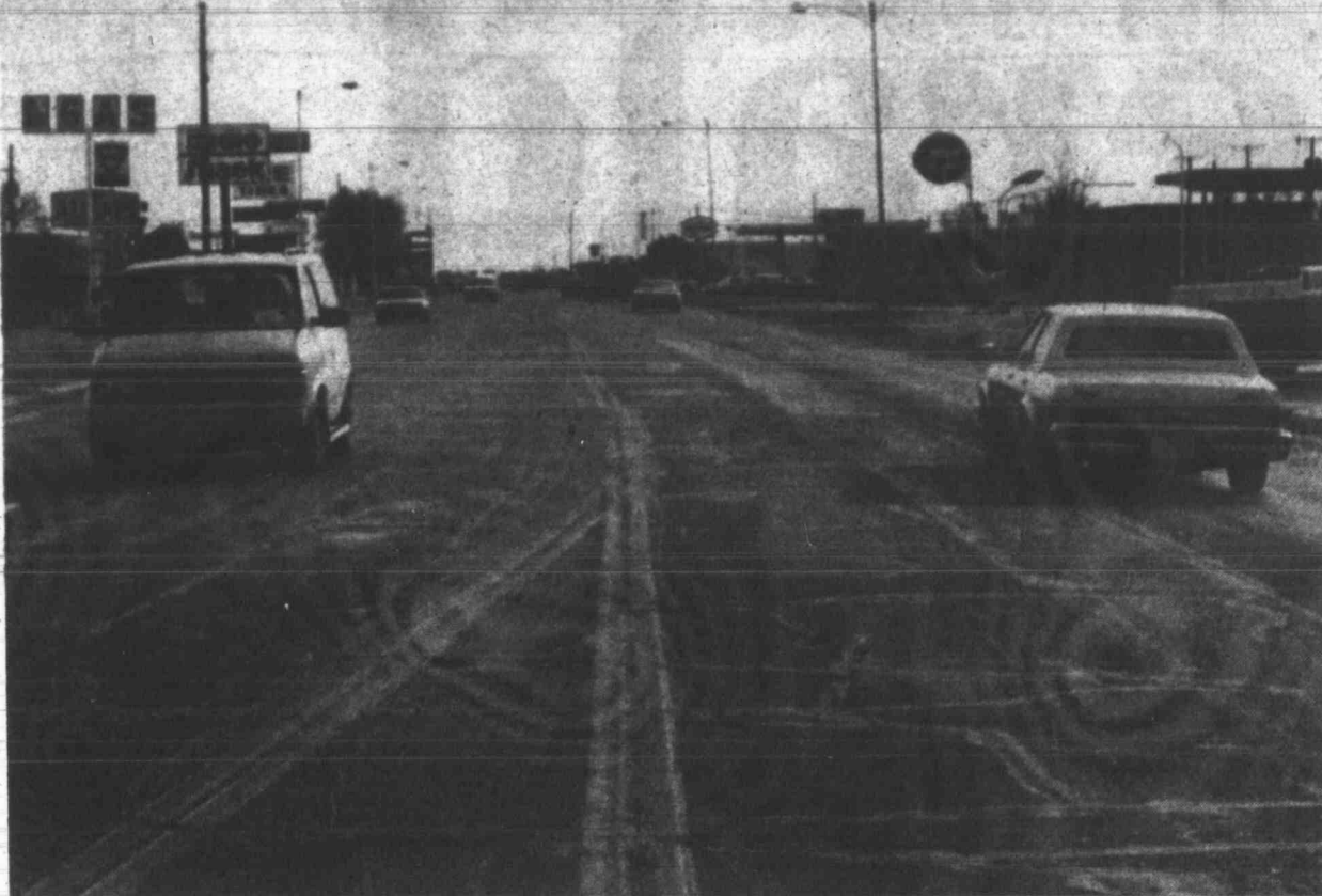
Above is shown a segment of Highway 70 in the Texas Panhandle community of Pampa that has been targeted for a proposed widening. The highway is a highly congested major north/south thoroughfare with a high traffic accident rate.
