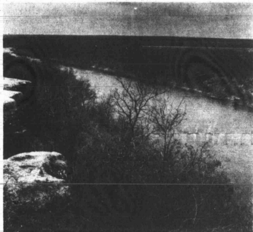
1987 represented a historic year for the Colorado River Municipal Water District, with construction work finally beginning on the Stacy Dam project, after a dozen years awaiting the permit. The scene at left is a view of the Colorado River, an area that will
