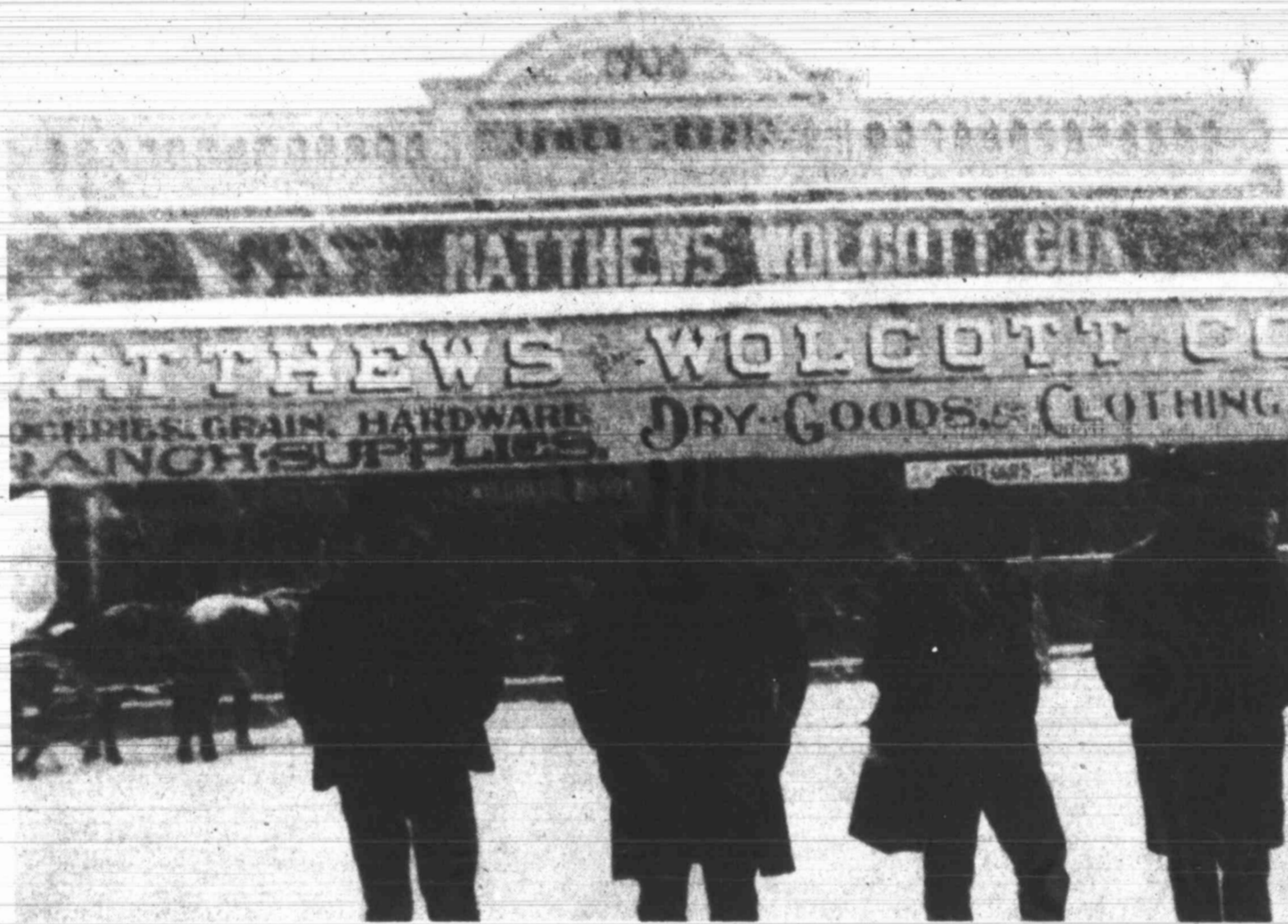
The Big Spring Hardware Company presently occupies this building, shown above in a 1903 photograph furnished by the Howard County Historical Commission's Polly Mays. The original belonged to Paul Soldan of Big Spring, who identified three of the four railroad men photographed in the snowstorm as, from right, Charles Ruhrup, railroad engineer Louis C. Soldan and Emil Farenkamp.
