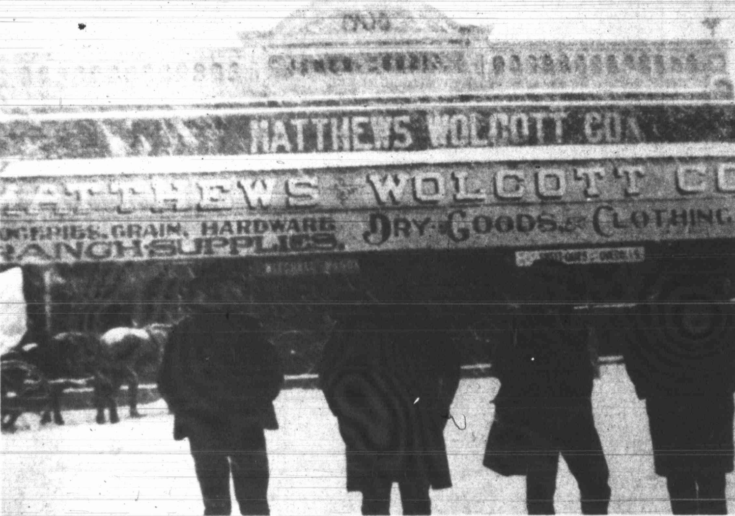
The Big Spring Hardware Company presently occupies this building, shown above in a 1903 photograph furnished by the Howard County Historical Commission's Polly Mays. The original belonged to Paul Soldan of Big Spring, who identified three of the four railroad men photographed in the snowstorm as, from right, Charles Ruhup, railroad engineer Louis C. Soldan and Emil Farenkamp.
