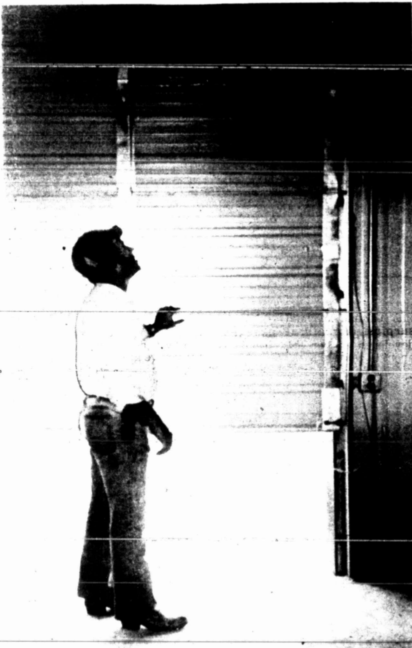
OVERHEAD DOORS — Reinert Welding & Steel Construction recently installed overhead doors for a storage building for the Big Spring Herald. Ralph Reinert, owner, is overseeing the installation.
