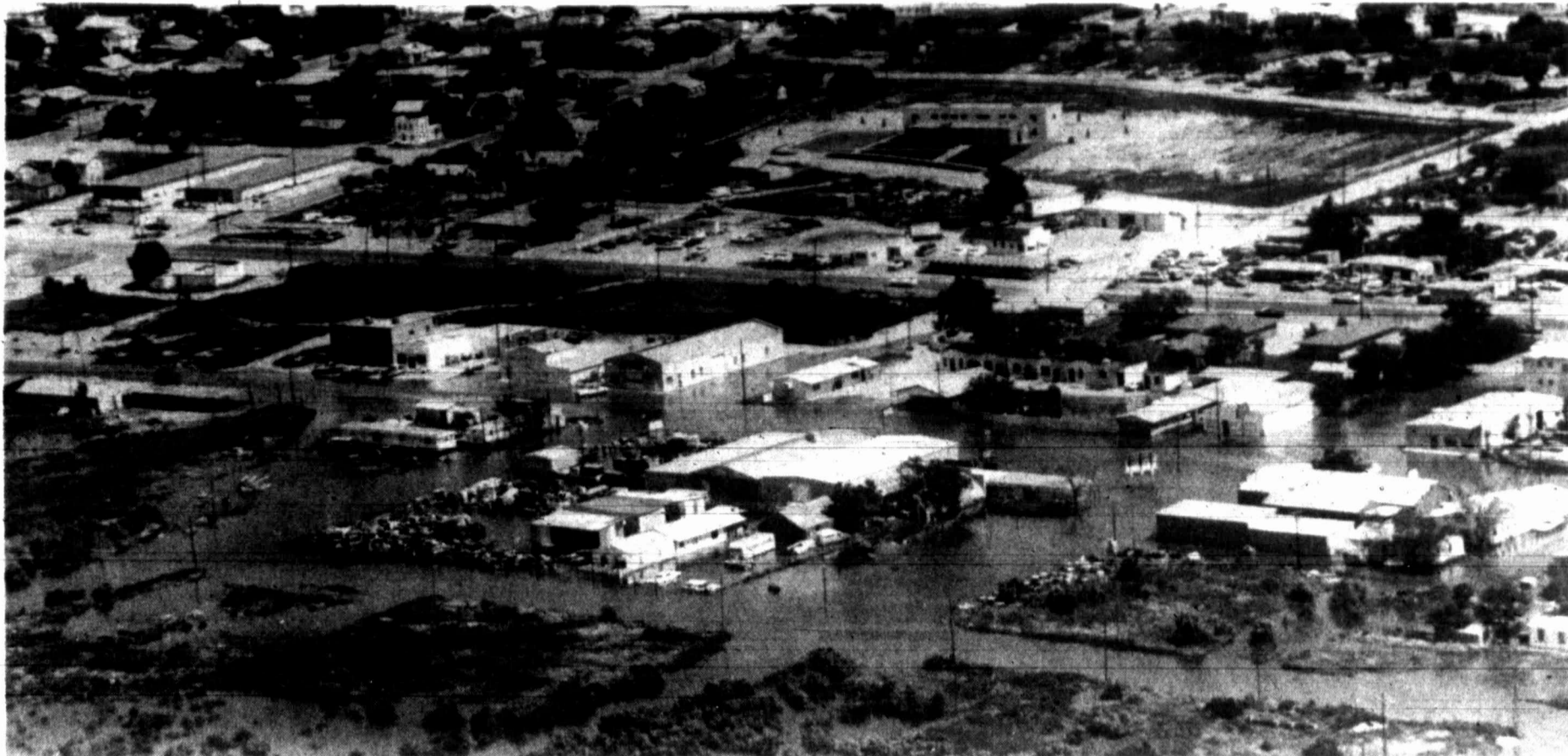
An aerial photograph of Jones Valley Thursday afternoon shows a view toward the southeast of the flooding in that area, as a result of runoff from Natural Dam Lake west of Big Spring. The area shown in the photograph in-
