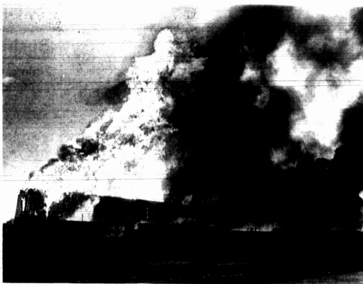
The ADM grain elevator in Burlington, Iowa, exploded into a giant fireball at approximately 10:40 a.m. Friday. Five people were reported to be injured and were taken to the hospital. Authorities were still unsure of the cause or outcome of the disaster Friday evening.
