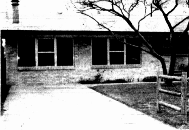
GARAGE CONVERSION — Reclaim all that valuable space now in your garage. When Bob's Custom Woodwork does the job, the staff carefully matches windows, materials and design (both inside and out) so that the conversion does not look like it's just been "added on." Pictured is an example of the firm's work.
