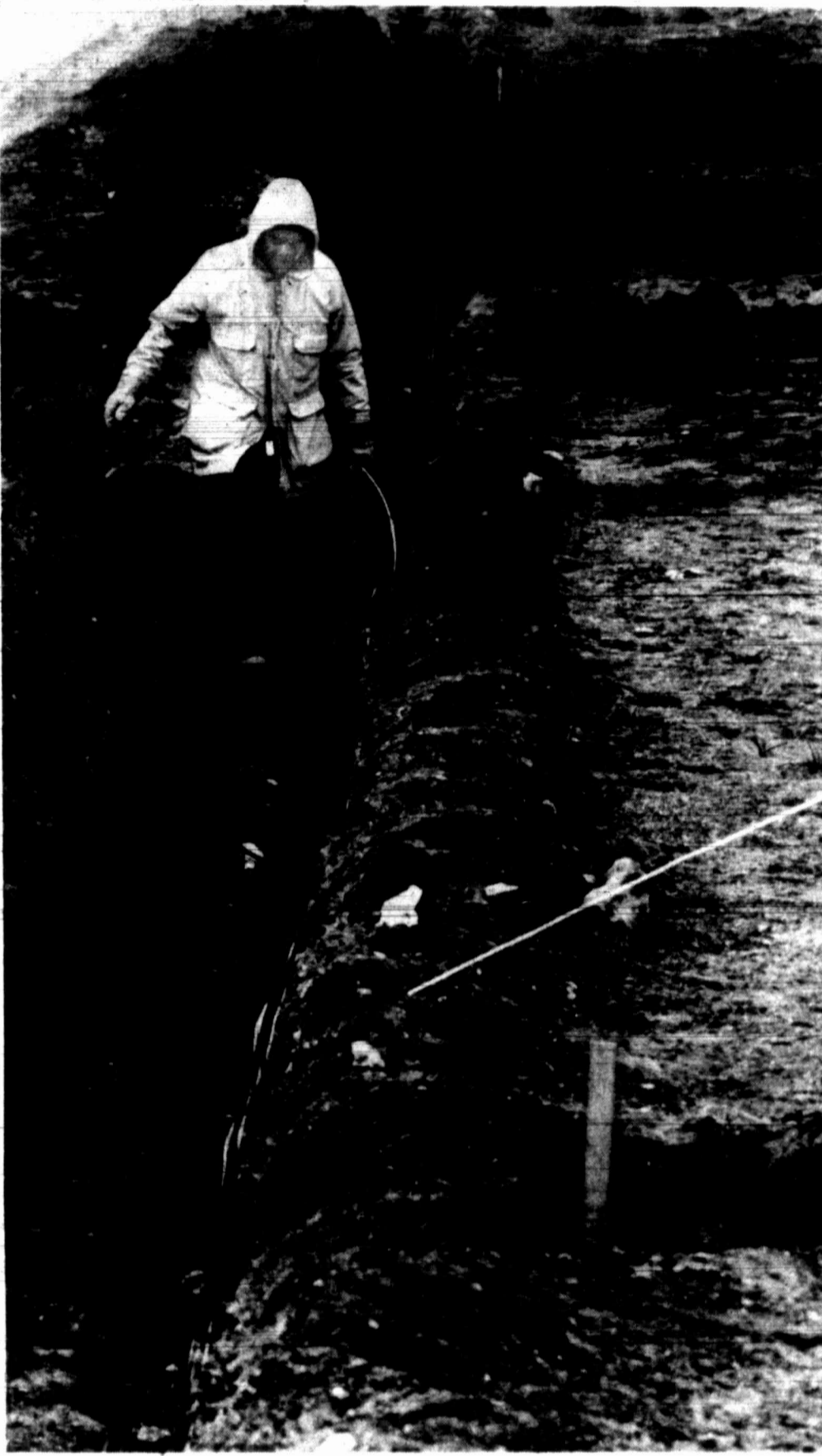
Big Spring Federal Prison Camp inmate Richard Schell lays a wire over the water line at Comanche Trail Park golf course Tuesday morning. The newly installed sprinkler system will be electronically controlled from the clubhouse.
